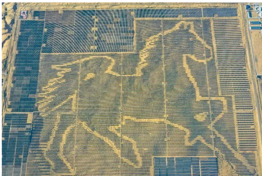
Fig. 2-4 The Horse-shaped Solar Power Station at the Kubuqi Desert, Inner Mongolia Autonomous Region
