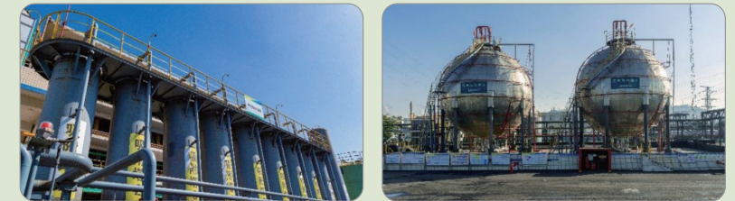
Figure 3. Chloromethane PSA unit and spherical tank (Credit: Fuhua Tongda Chemical Co., Ltd.)
