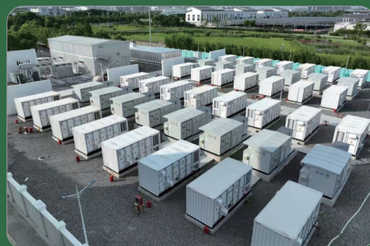
Figure 1 50 MW / 100 MWh Grid-side Energy Storage Project of Suzhou Shengneng (Credit: Energy Foundation China)
